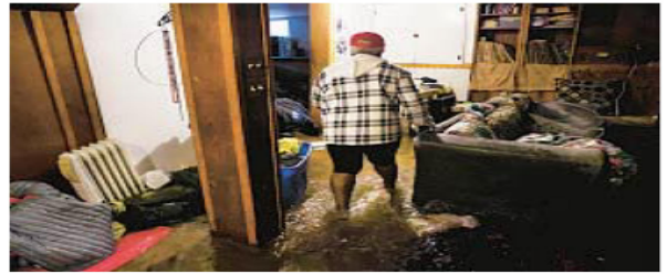
Shirley Howard stands in her flooded basement in the 800 block of North Lockwood Avenue on Sunday in Chicago's Austin neighborhood amid weekend thunderstorms that sparked flash flood warnings. STACEY WESCOTT/TRIBUNE
