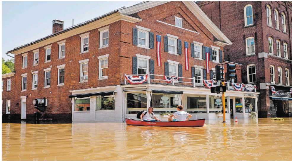
Flooding in Montpelier, Vt. The lack of a national rainfall database and of up-to-date flood maps hamper preparations for major storms.
