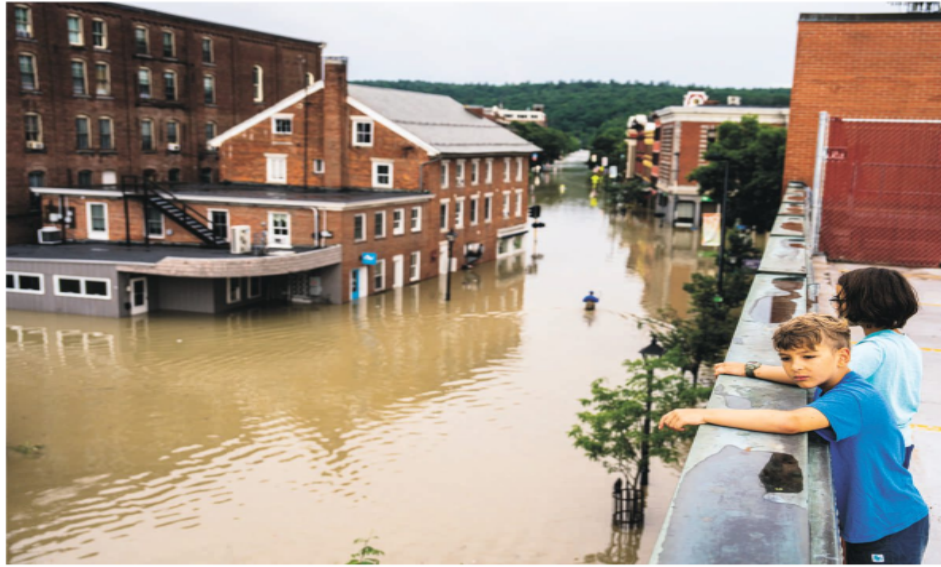
Streets in downtown Montpelier, Vermont's capital, were underwater after intense storms that started Sunday brought six to nine inches of rain to certain areas. The search for people stranded by flooding in the rural, mountainous state was expected to take several days.
