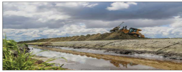
A DARK BAND of liquid, top, spreads within the floodwaters of Tulare Lake in Corcoran, Calif. Above, an earthmover forms a makeshift levee wall beside a swelling irrigation ditch at the lake.
